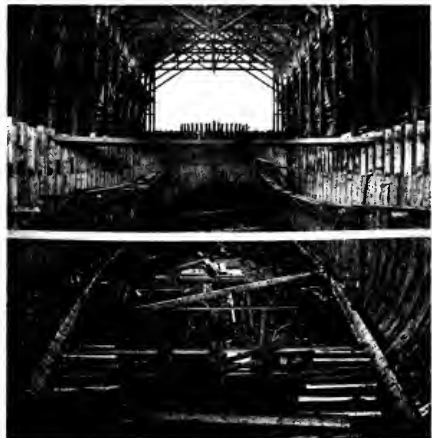
Interior view of the framing of the "Anyox."
